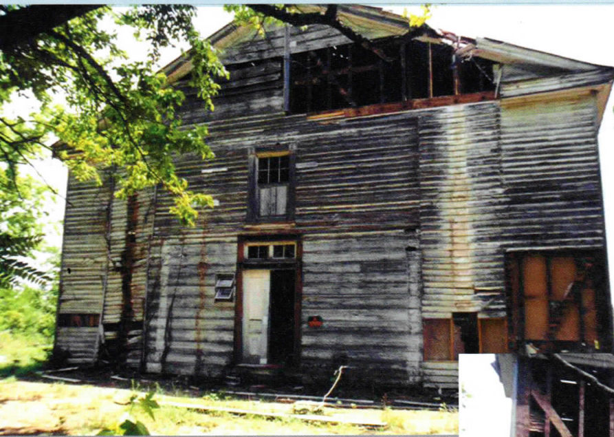
Unusual ca. 1840 house with dual gable end chimney facades
